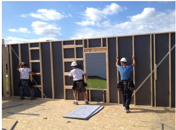
**Above:** Tim O'Brien Homes builds the new HP+ High Performance Wall System showing the BASF Neopor®, a graphite-enhanced rigid foam insulation sheathing that is stronger than a typical new home.
